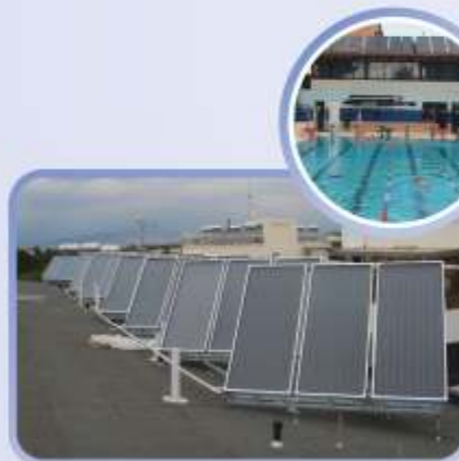
On roof installation
