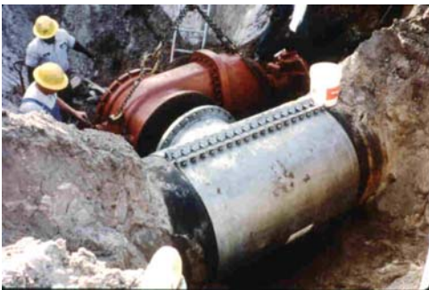
Tapping sleeve on distribution pipe
