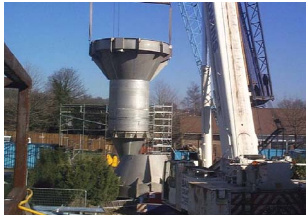
Installation of complete water softening reactor
