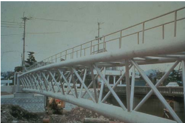
Bridge to carry drinking water across river, Tokyo, Japan
